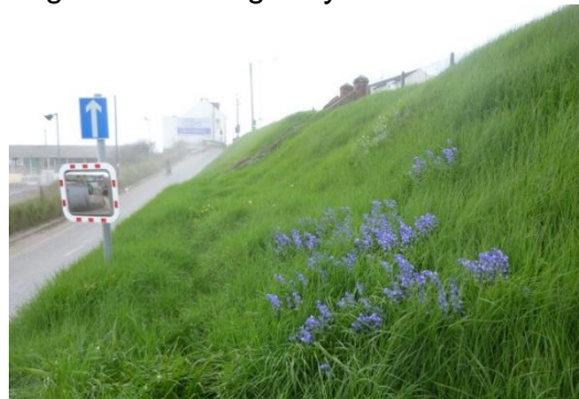
Basin Road North embankment
